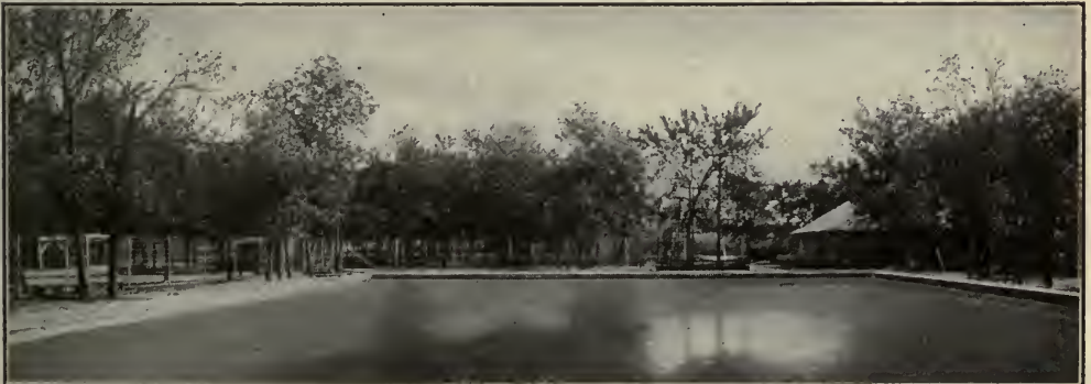
CONCRETE SWIMMING POOL BUILT WITH WHITE WATER-PROOF CEMENT, HASTINGS, NEBR.
